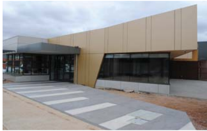
CRC Melton - Engineering
