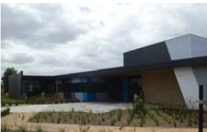
Victoria University SC Tele-Communication / Cabling Plastering Painting & Decorating Refrigeration & Air Conditioning
